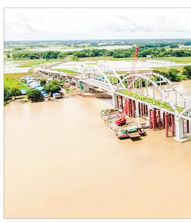
Kyunpyathat Bridge is a steel box girder with the floor of reinforced concrete and can withstand up to 60 tones of weight.—(Photo: IPRD)
