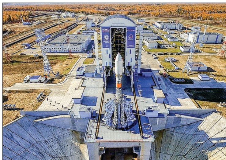
The first stage of the work to fix cavities detected under the casing of the launch pad at the Vostochny Cosmodrome has been completed. PHOTO: TASS
