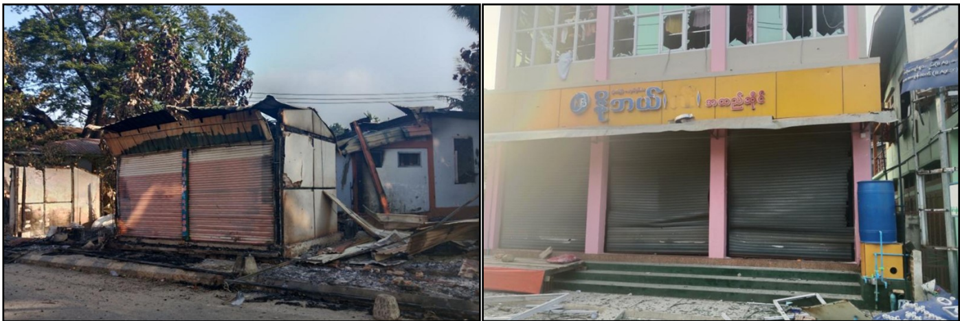
Damages of residential houses and departmental buildings in the terrorist acts of the KIA group and the so-called PDFs
