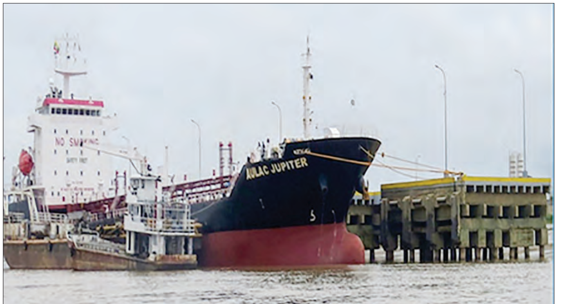
Photo shows the Green Asia Port Terminal (Thilawa)
